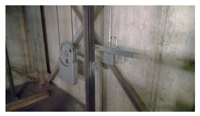
Figure 2-8: Encoded Tape Mounting – Bottom Bracket
