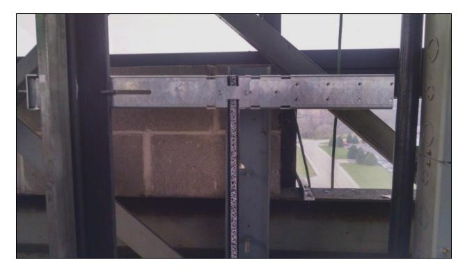
Figure 2-2: Encoded Tape Mounting – Top Bracket
