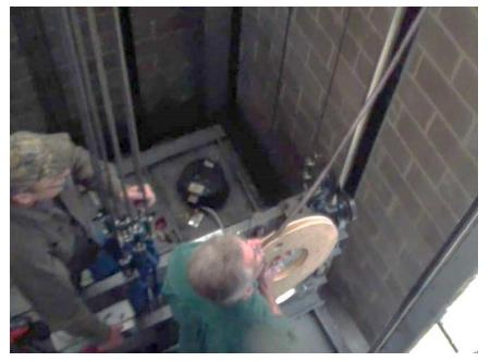
Figure 2-5: Unroll the Encoded Tape
